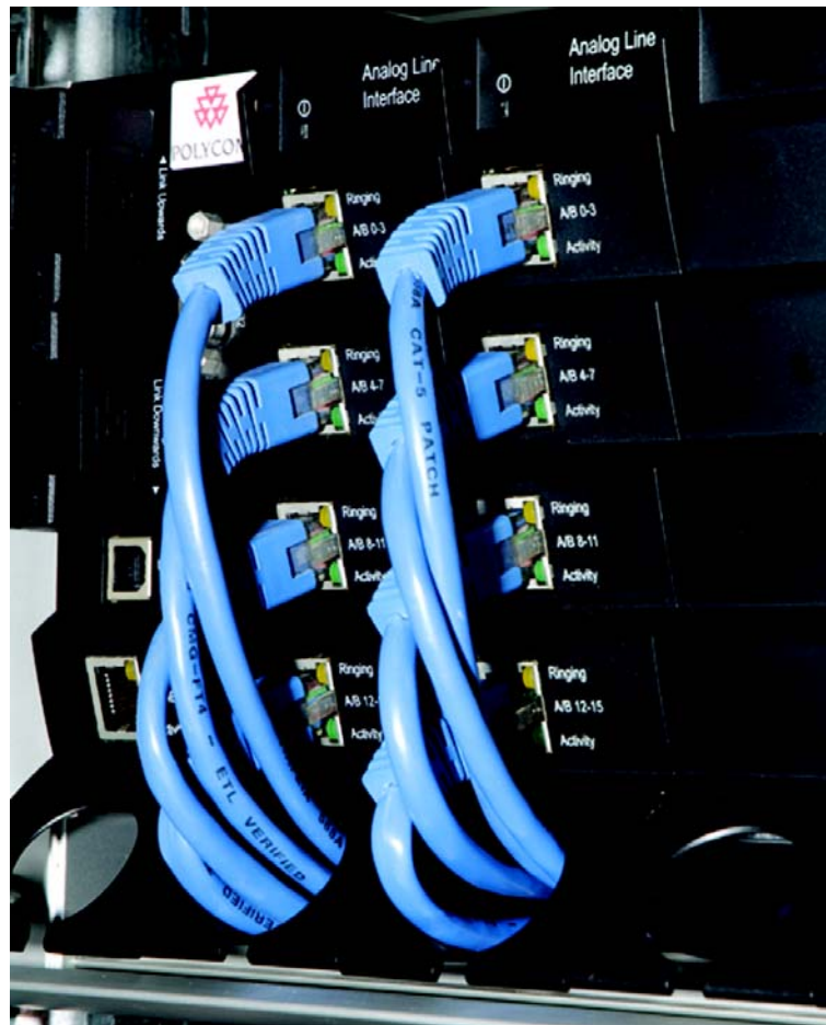
Figure 10 Harnessing cables to the back and out
