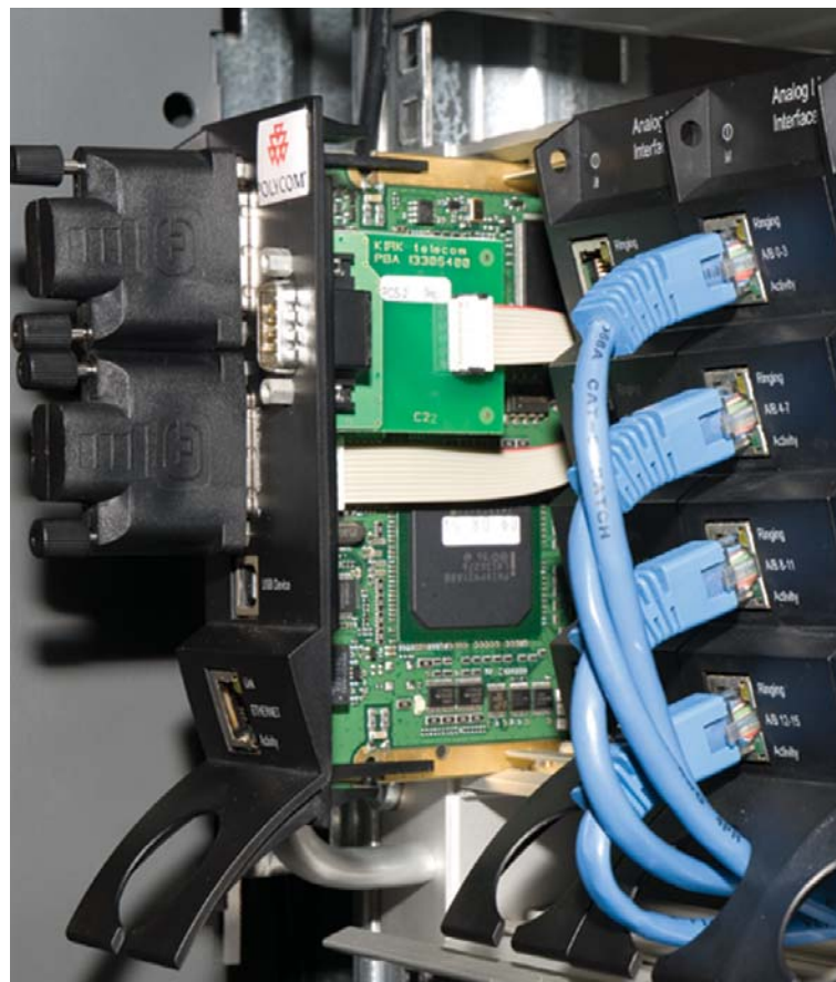
Figure 10 Installing CPU card
